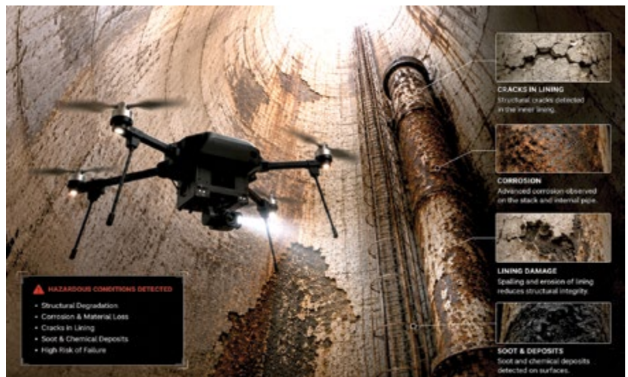
Inspecting the interior of an industrial chimney to identify structural damage and potential hazards before personnel enter
